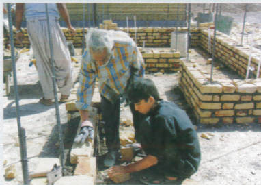
A model house with an earthquake-resistant structure under construction.
