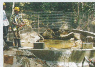
Constructing waterworks utilizing the gravity water supply system.
